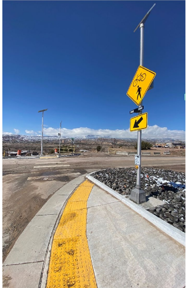
Figure 42. Image. RRFB Crossing located at the Intersection of Bear Head Canyon Road and NM-4.
