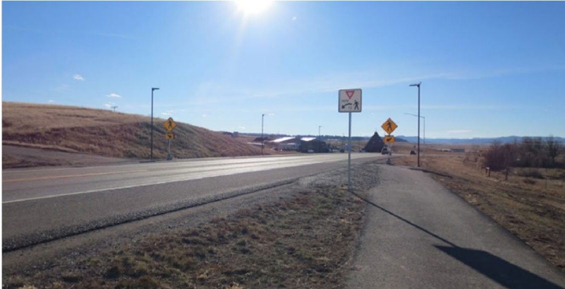
Figure 34. Image. A pedestrian crossing with RRFB signs was installed on Highway 212 in the south Busby, MT, community.
